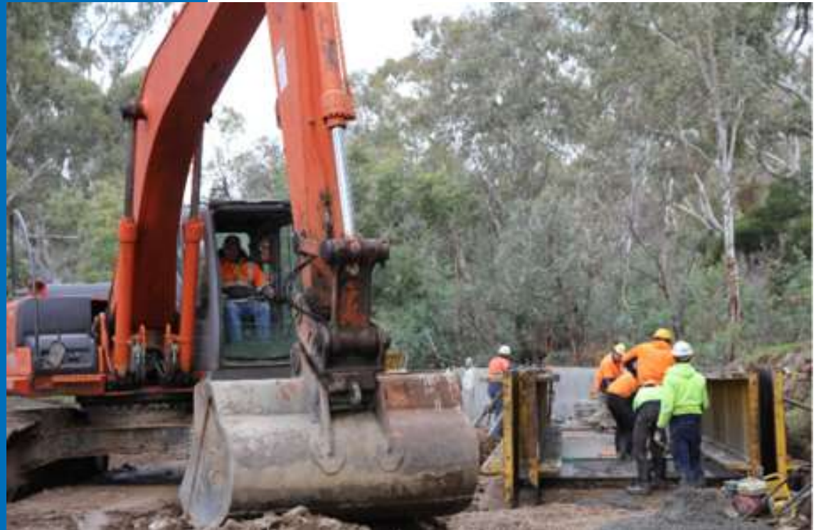
Coliban Main Channel Renewal Project – Credit: Coliban Water.
